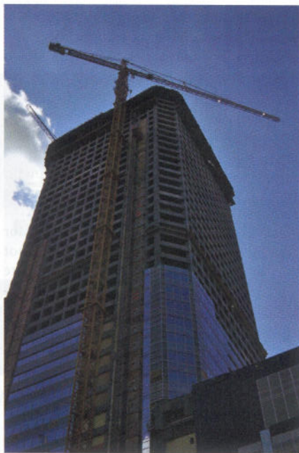
A Liebherr 550 EC-H 20, a 630 EC-H 20 Litronic and an Alimak FC6800-12D HS are used by Batson-Cook Company in Charlotte, NC on the Wachovia (BOA) Center
